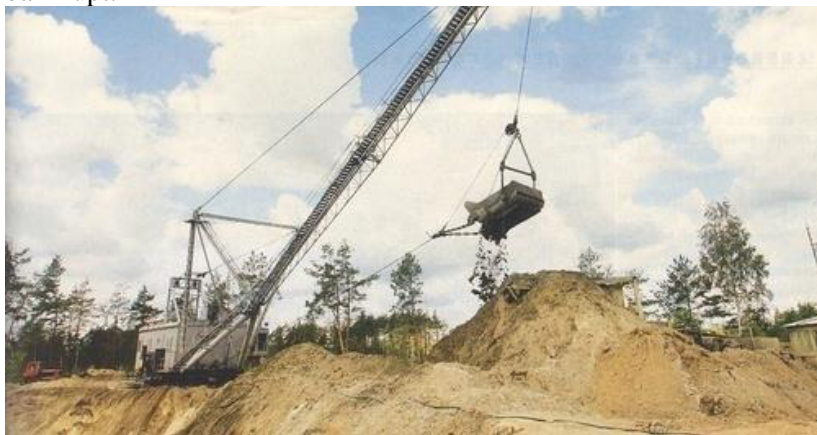
Fig. 5. Preparation of the massif for extraction of amber in the quarry by excavation method
