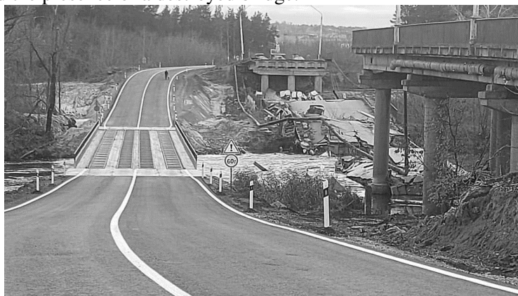
Fig. 2. Temporary bridge across the Siverskyi Donets River (Izyum, Kharkiv Region) [6]
