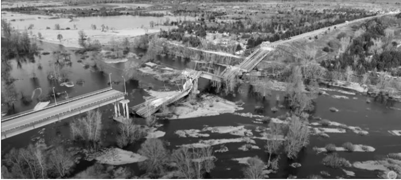
Fig. 3. The destroyed bridge over the Dnipro River. Frame from the movie “RIK” (“The Year”, 2023) [7]
