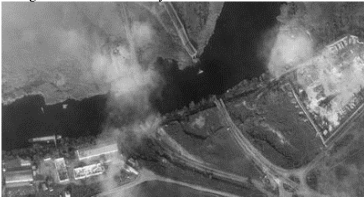
Fig. 4. The destroyed Darivskyi road bridge across the Ingulets River (Kherson Region) [8]
