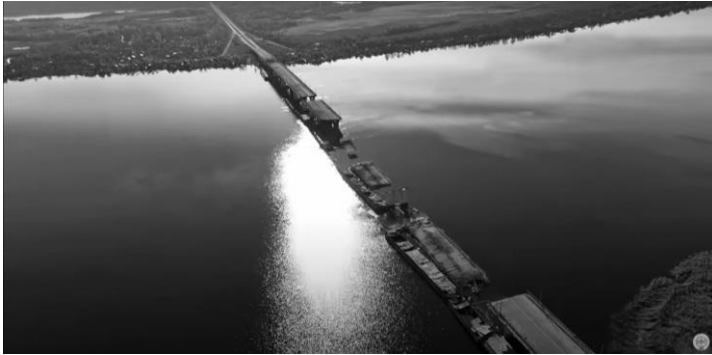
Fig. 5. The ruined Antoniv bridge across the Dnipro River Frame from the movie “RIK” (“The Year”, 2023) [9]
