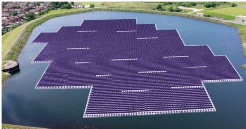
Fig. Example of solar panels placement: South Korean company Solkiss plans to install a floating solar power plant on the Deoku reservoir. The capacity of the power plant will be 2,67 MW
