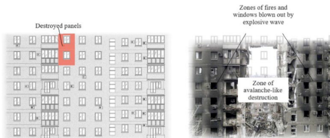
Fig. 6. Nature of damage and scheme of destruction of a panel building in the city of Mariupol
