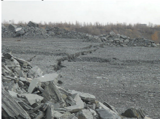
Fig. 1. Scheme of forming cracks on the northern side of the Open Pit No 1 of the Mining and Processing Plant “Novokryvyi Rih GOK”(formation of terraces)
