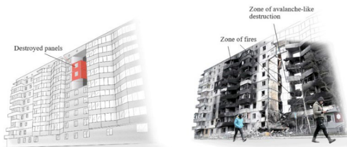
Fig. 5. Nature of damage and scheme of destruction of a panel building in the town of Borodyanka
