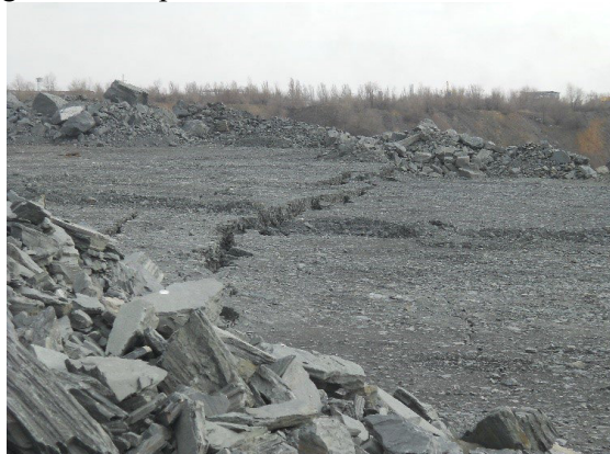
Fig. 1. Scheme of forming cracks on the northern side of the Open Pit No 1 of the Mining and Processing Plant “Novokryvyi Rih GOK”(formation of terraces)
