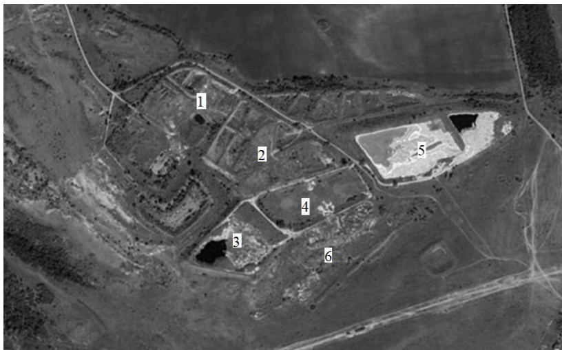
Fig. 3. The industrial site of the landfill
