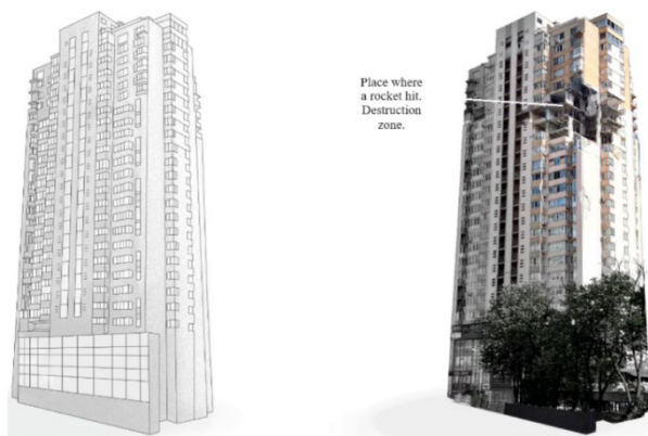
Fig. 11. Nature of damage to a multi-story building with a reinforced concrete frame
