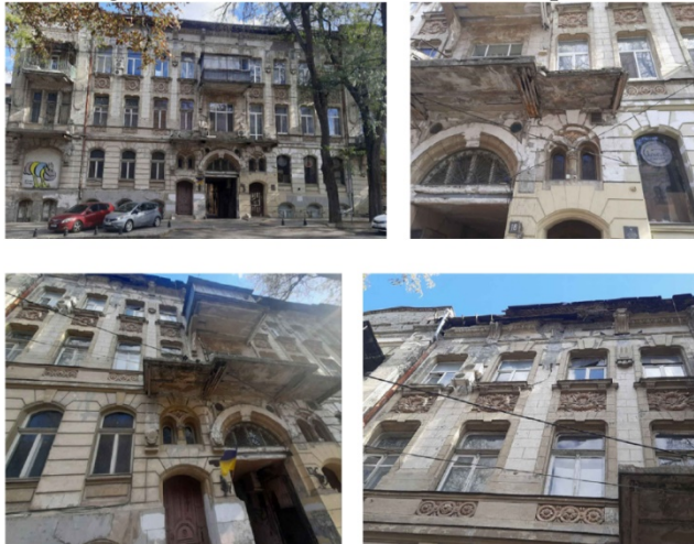
Figure. Photographic recording of the condition of the facade elements
